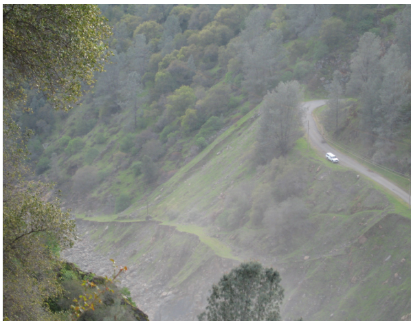
View south from Englebright Dam
