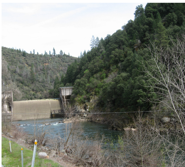
Chili Bar Dam looking east
