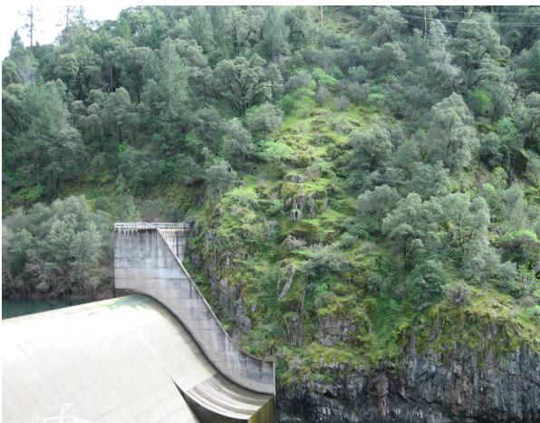
Chili Bar Dam (looking south)
